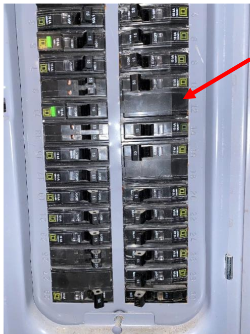
2d: - medium shot all your breakers and if you have any open slots for future breakers for the solar back-feed
