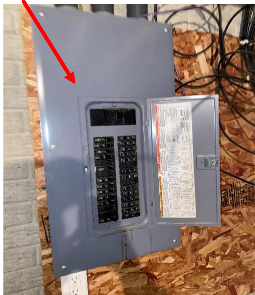
2d: - medium shot all your breakers and if you have any open slots for future breakers for the solar back-feed
